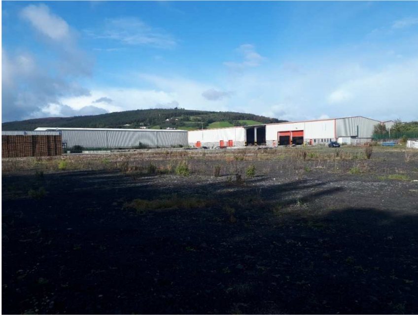
Photograph 3.3. Looking north and west.
