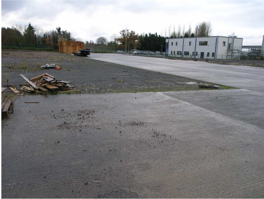
Figure 11.10: Existing concrete surface along west and north side of the development area (looking east)
